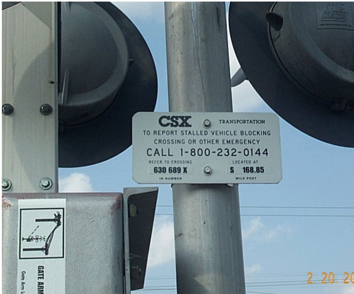
Photograph provided courtesy of Mr. Ric Cruz, Crossing Inventory Engineer, NC Department of Transportation.
